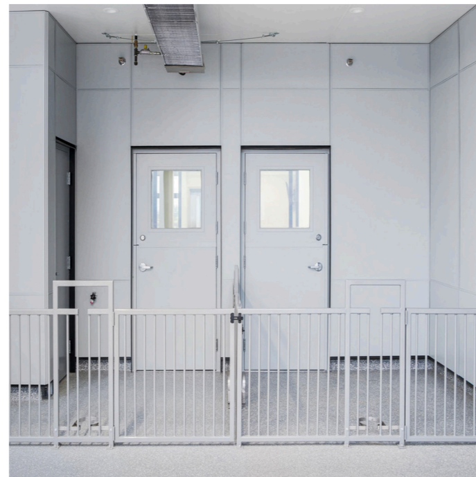
Neonatal Nursing Station exterior
